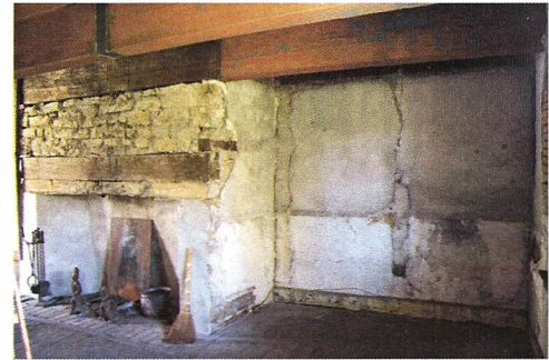
Fireplace, Bar Area before (R.Burch)
