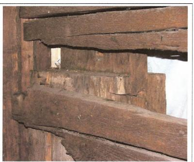
two-story frame, the original corner post was not load bearing, so it never was ended-out.
